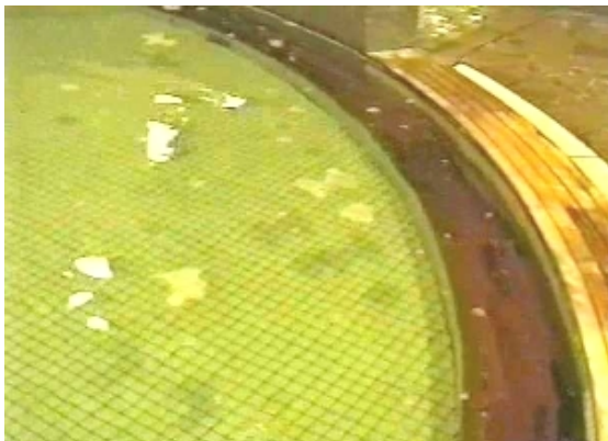
Biofilm removal started within hours after MIOX system start-up
