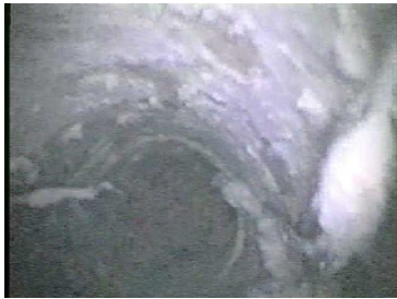
Feed water pipe with sodium hypochlorite
